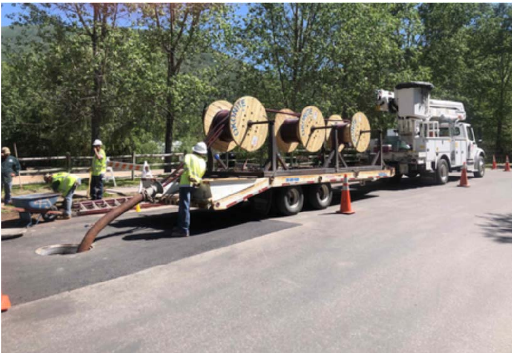
Sturgeon Elec. Feeding new electrical cables
