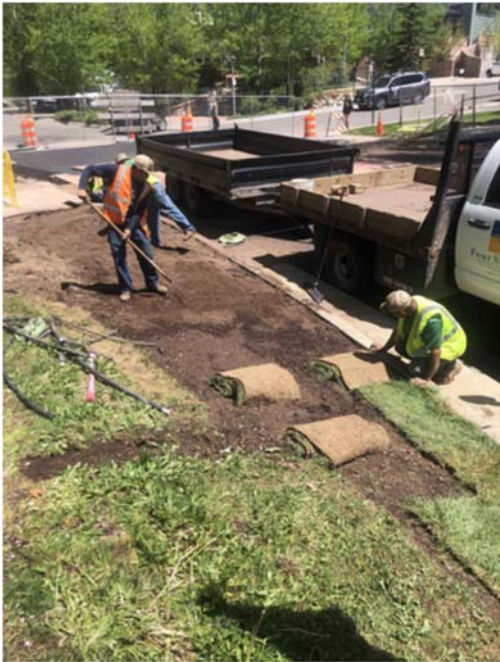
New sod patches being installed
