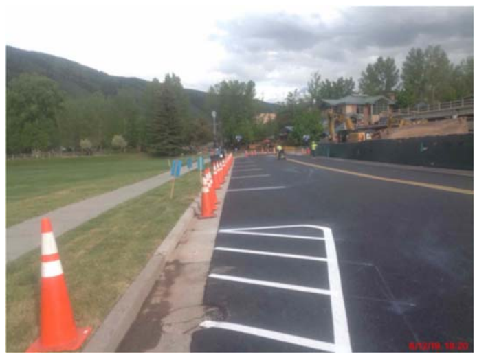
Striping being applied to new road surface
