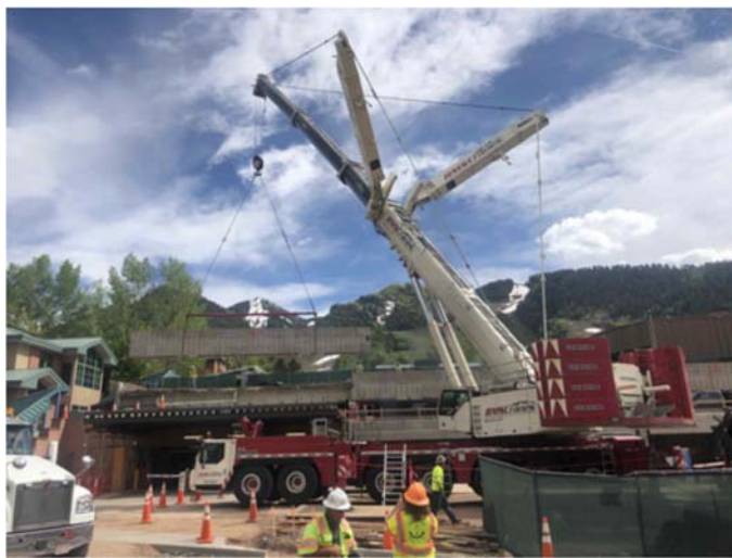
Crane pick of first beam
