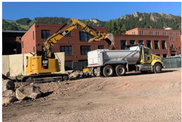
Removal of soils off site from initial 4' excavation of building foundation
