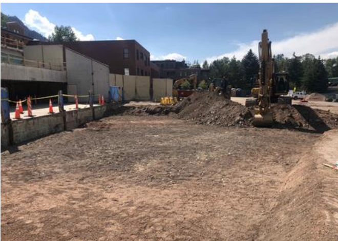
Beginning of the foundation excavation
