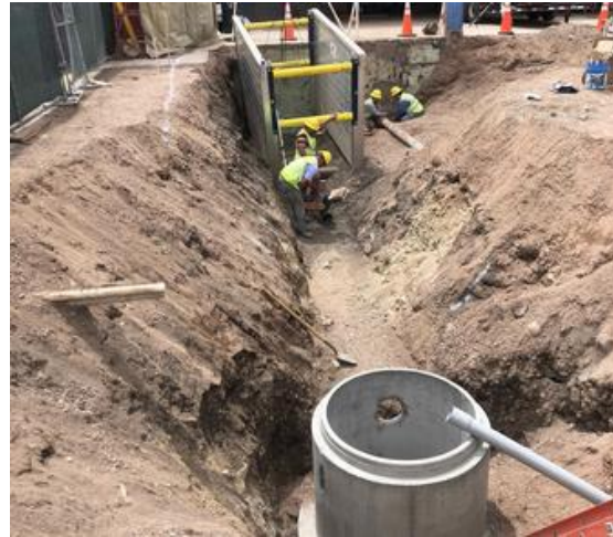
Rerouting of existing storm drain
