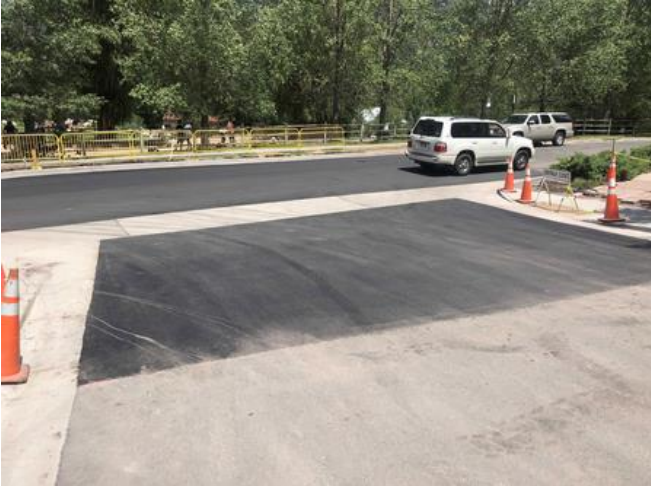
Asphalt paving complete at RGP & Founders Pl.
