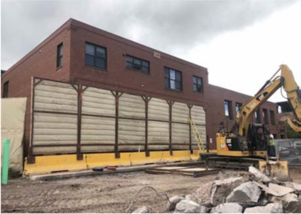
Sound wall at SW building corner
