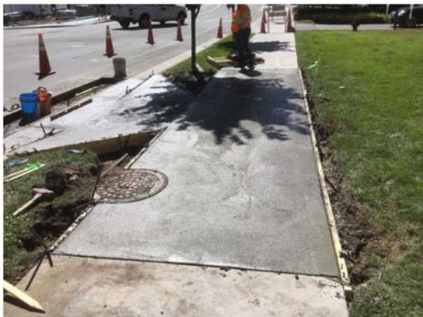
New ADA ramp and sidewalk section at W Mill St.
