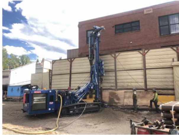
Drilling of front row vertical pipe piles
