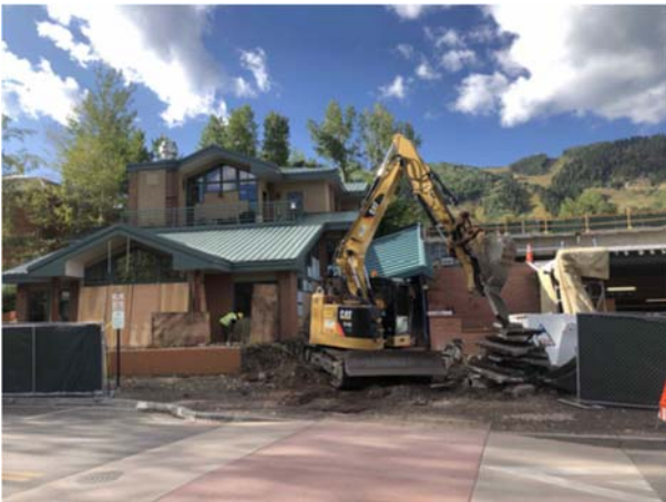
Beginning of stair and patio demo
