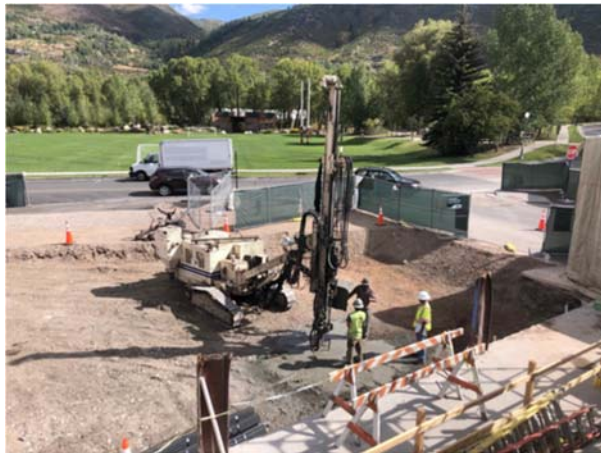
Placement of foundation micropile for pull testing
