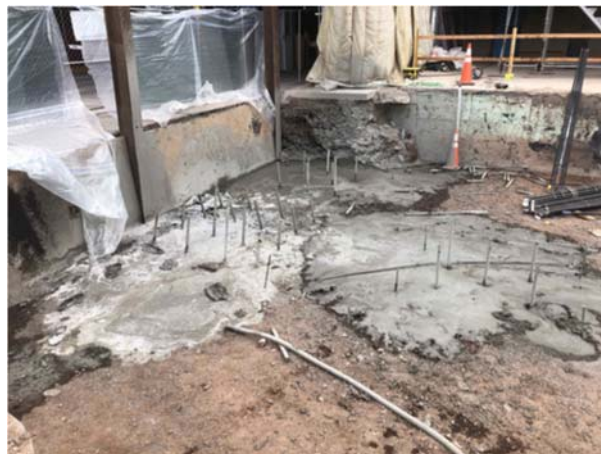
Foundation micropiles completed for two footings
