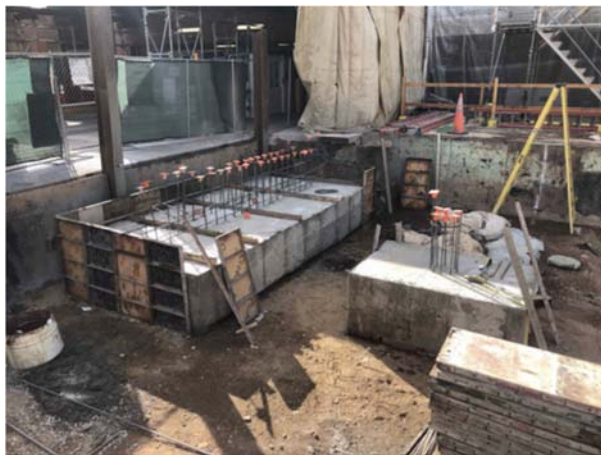
Foundation micropile cap footings
