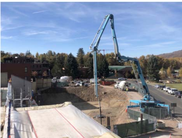
Concrete being pumped for the micropile footings
