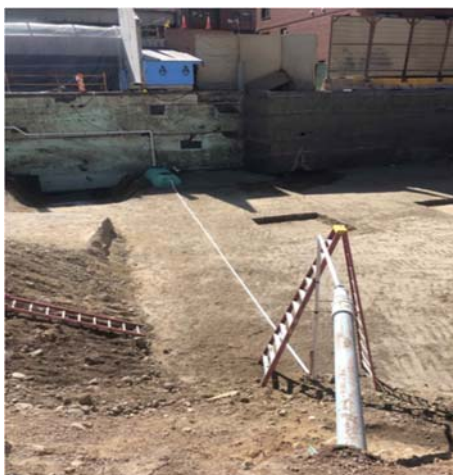
Temporary Sanitary Pipe
