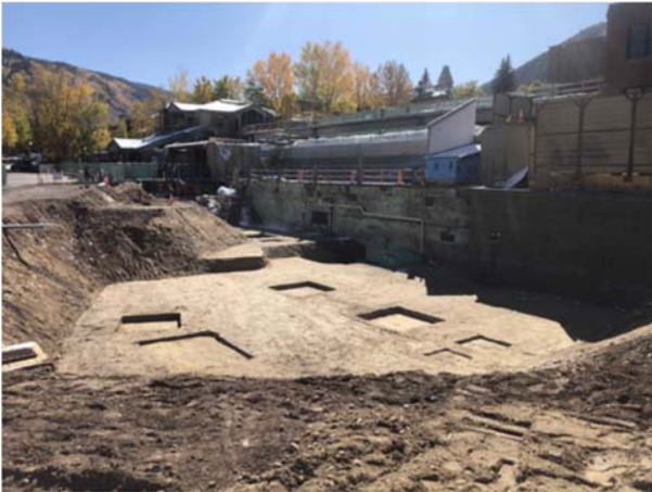
Excavation complete for Basement foundation
