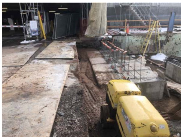
Backfilling at foundation micropile footings
