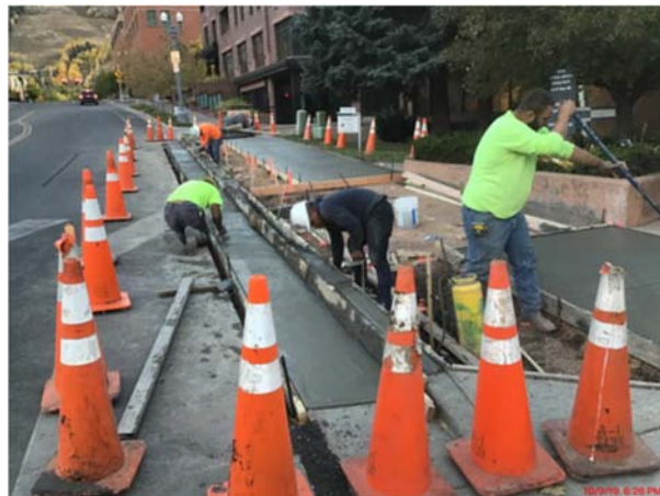
W. Mill St. Sidewalk and Curb and Gutter
