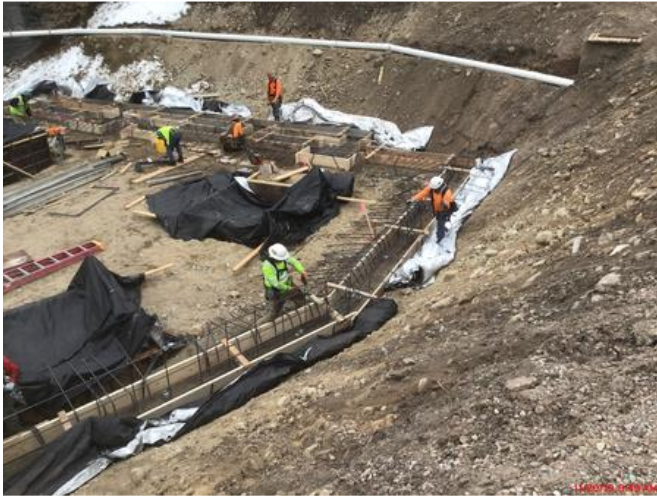
Placement of footing rebar
