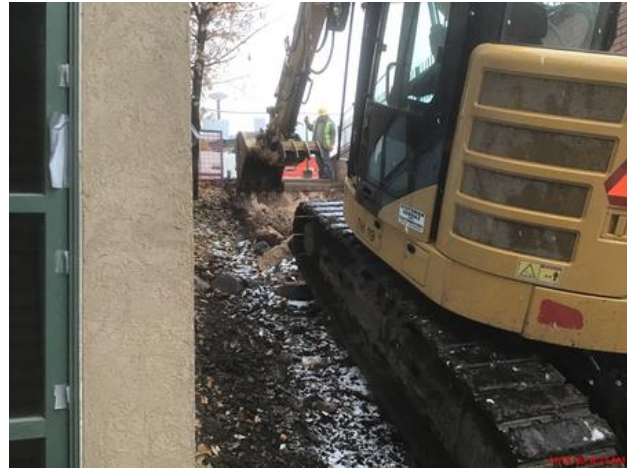
Upper level Grande stair demo
