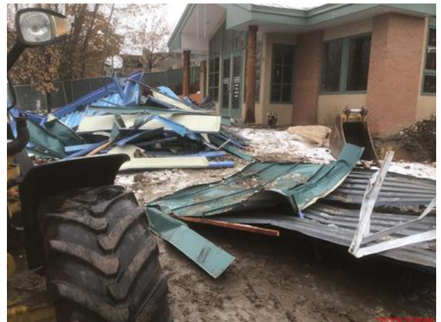
Stair Canopy Demo Debris
