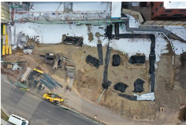
Arial view of foundation progress
