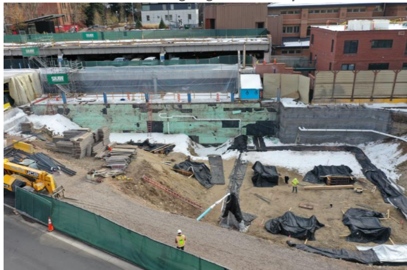
Arial view of foundation progress
