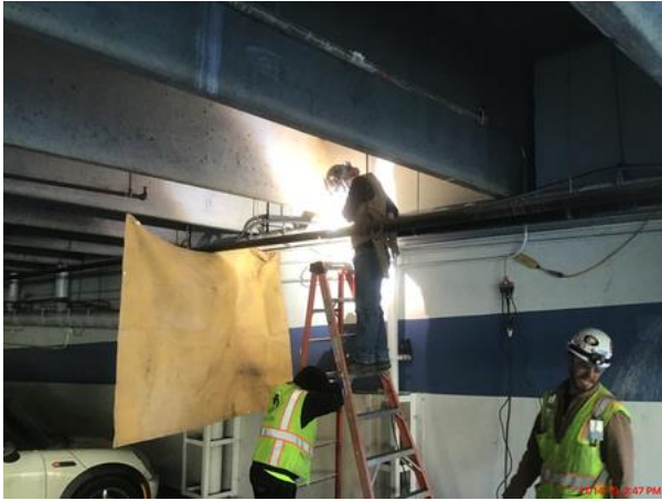
New gas line connection
