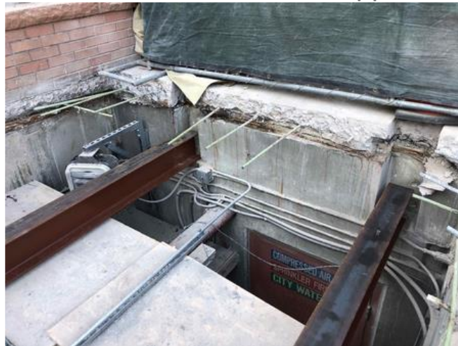
New beams at garage water entry deck
