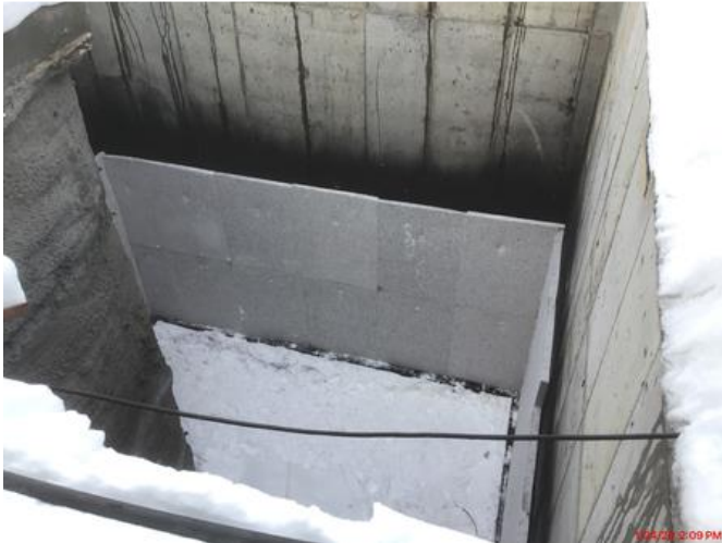
Foundation insulation
