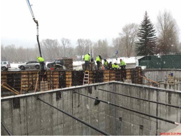
Placing foundation walls along GL 11
