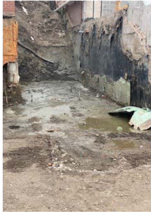
Rio Grande Elevator shoring installed
