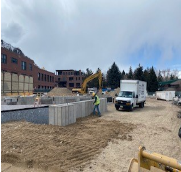
Foundation Backfill
