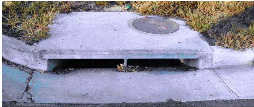
Figure 4.10.b Curb Opening Inlet
