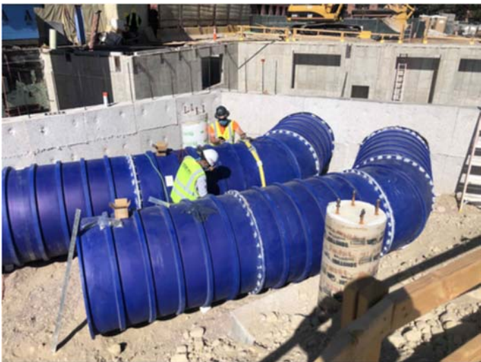
Underground duct
