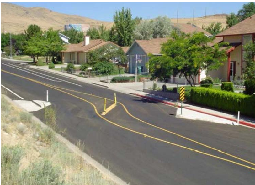
Figure 3 – Lateral shift example, City of Sparks Public Works: Traffic Division, Reno, NV
